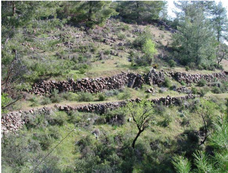
Figure 4.6: Structurally terraced Road Unit using rounded stone.
