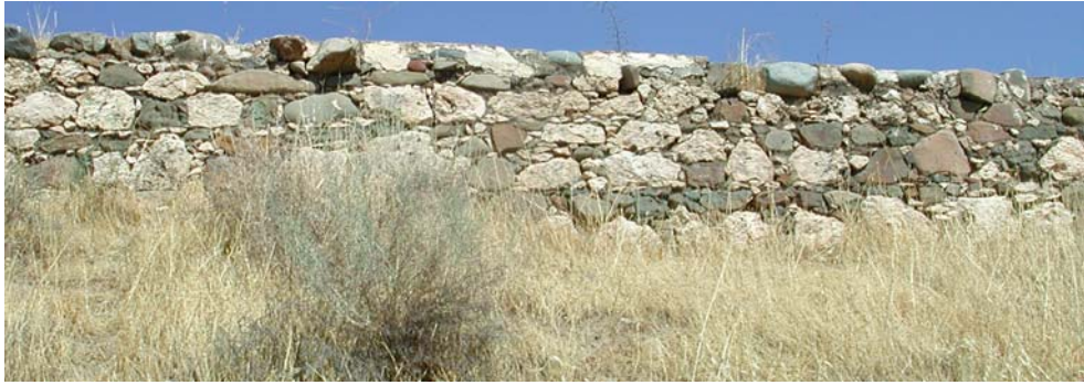
Figure 5.10: View of retaining wall on British Colonial road [DSCN0695]
