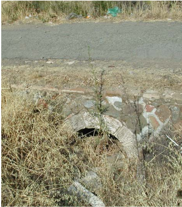
Figure 5.12:View of British Colonial period culvert in Road Unit RU0610 [DSCN0746]
