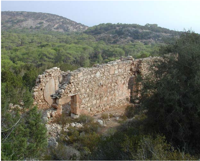
Figure 6.10: P024 Neochorio Magnesia structure showing substantial use of ashlar masonry especially around lintels and doorways.
