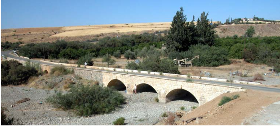
Figure 5.13: Eloea River Bridge at Kato Koutraphas Mandres (photograph taken by Chris Parks – TAESP)
