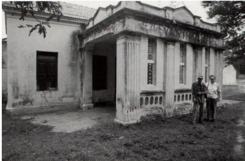
Fig. 5.26 Joubert Van Ingen and Pat Morris's wife outside 'the works' in 2003 © Pat Morris
