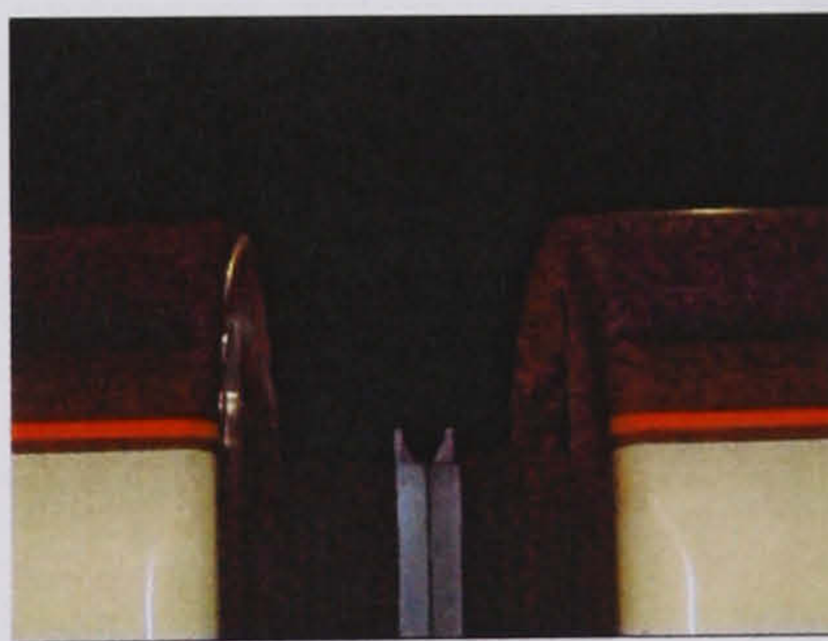
b. An Inter-car gap with protrusion evident on the cavity floor.
