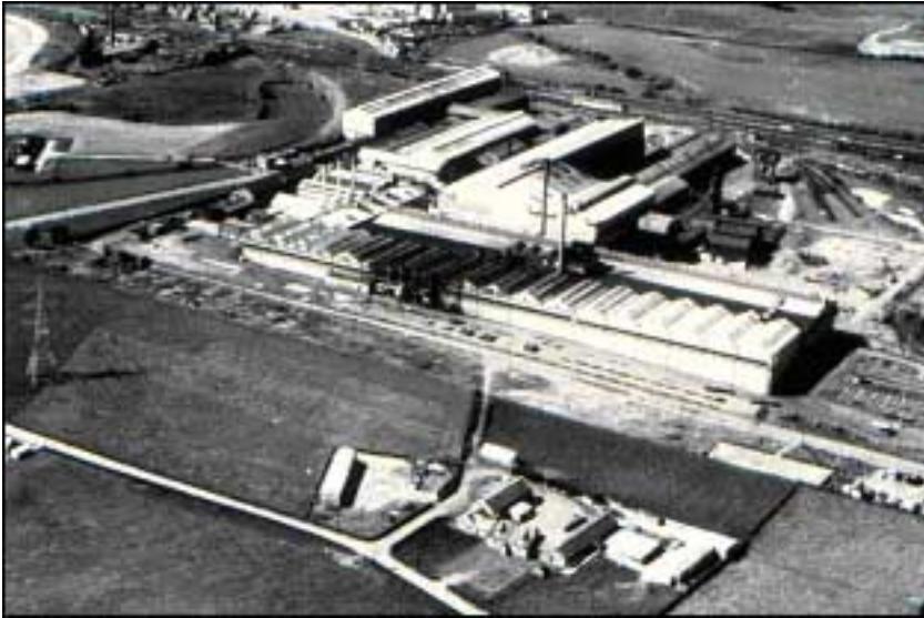
Figure 2.1 The Hallside Steelwork in its Heyday
