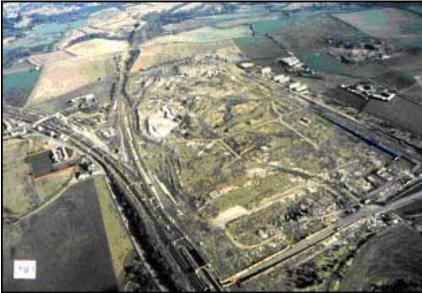
Figure 2.2 The Hallside Steelwork Circa 1995
