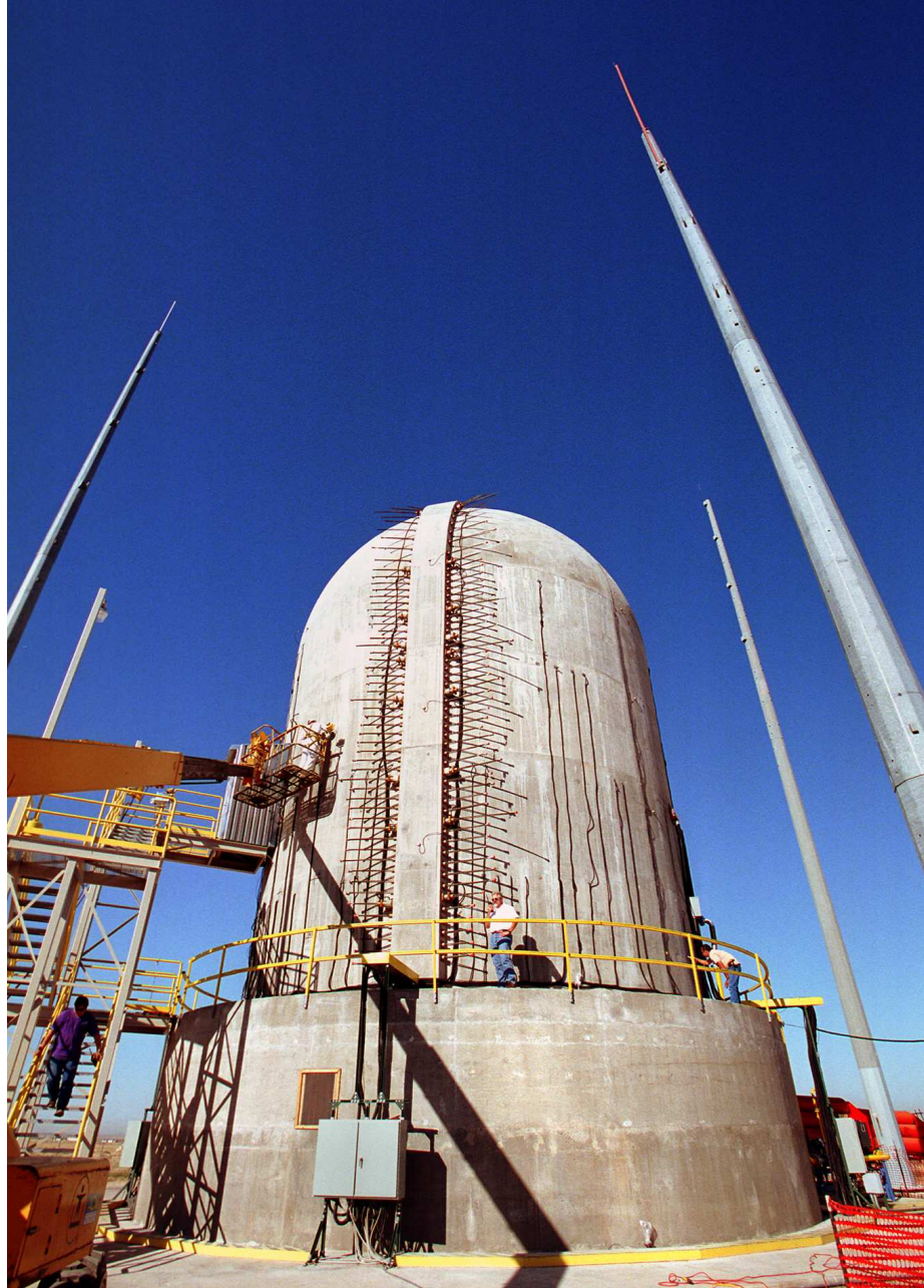
Figure 7.25.: Sandia National Laboratories test of a 1/4-scale model of a prestressed concrete containment vessel (PCCV) at an operating nuclear power plant in Japan.
