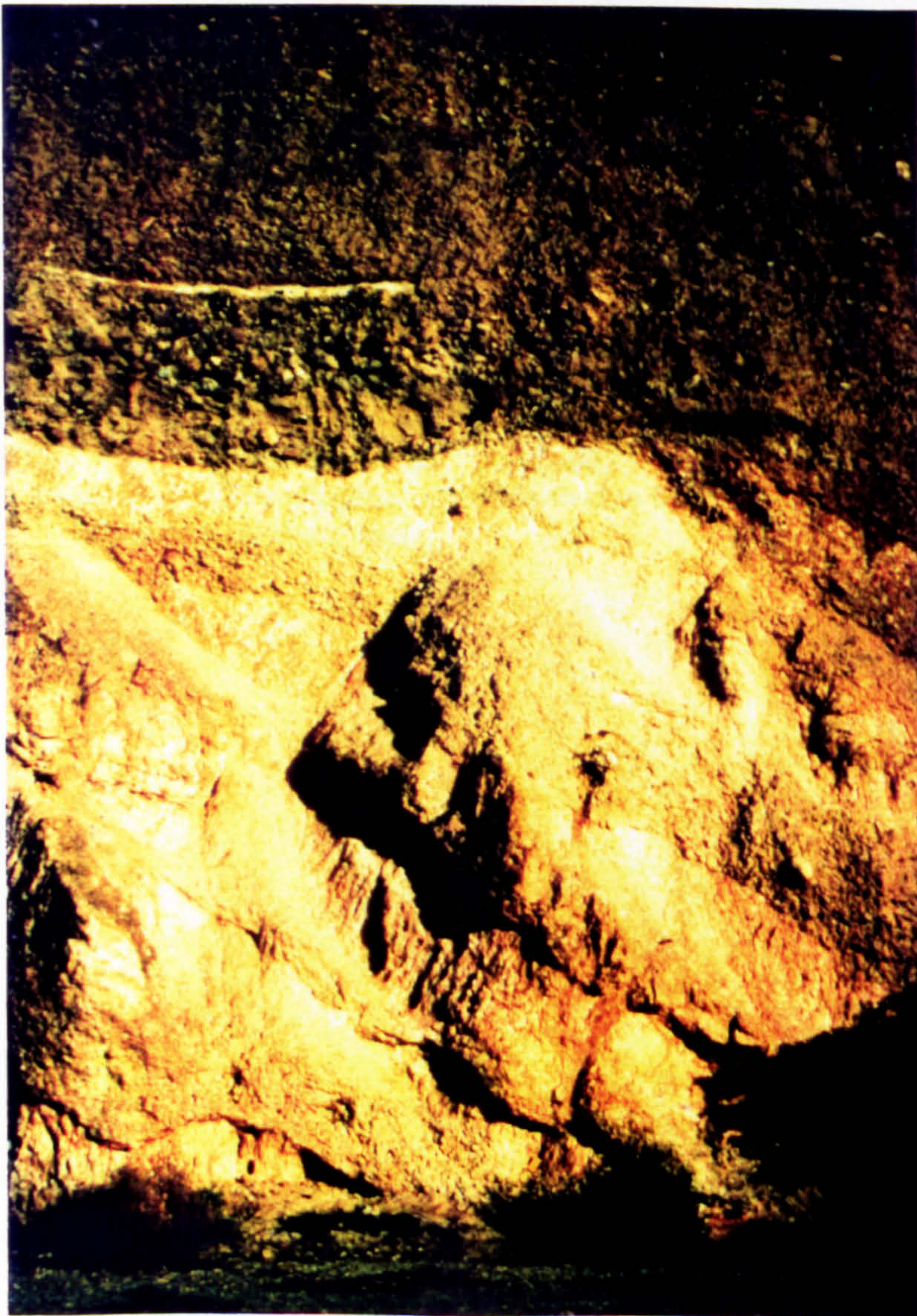
Fig. 7.15. Angular unconformity between the Shihr Group below and the Pliocene deposits in the Ad-Deis area to the south of wadi Kharid, looking east.
