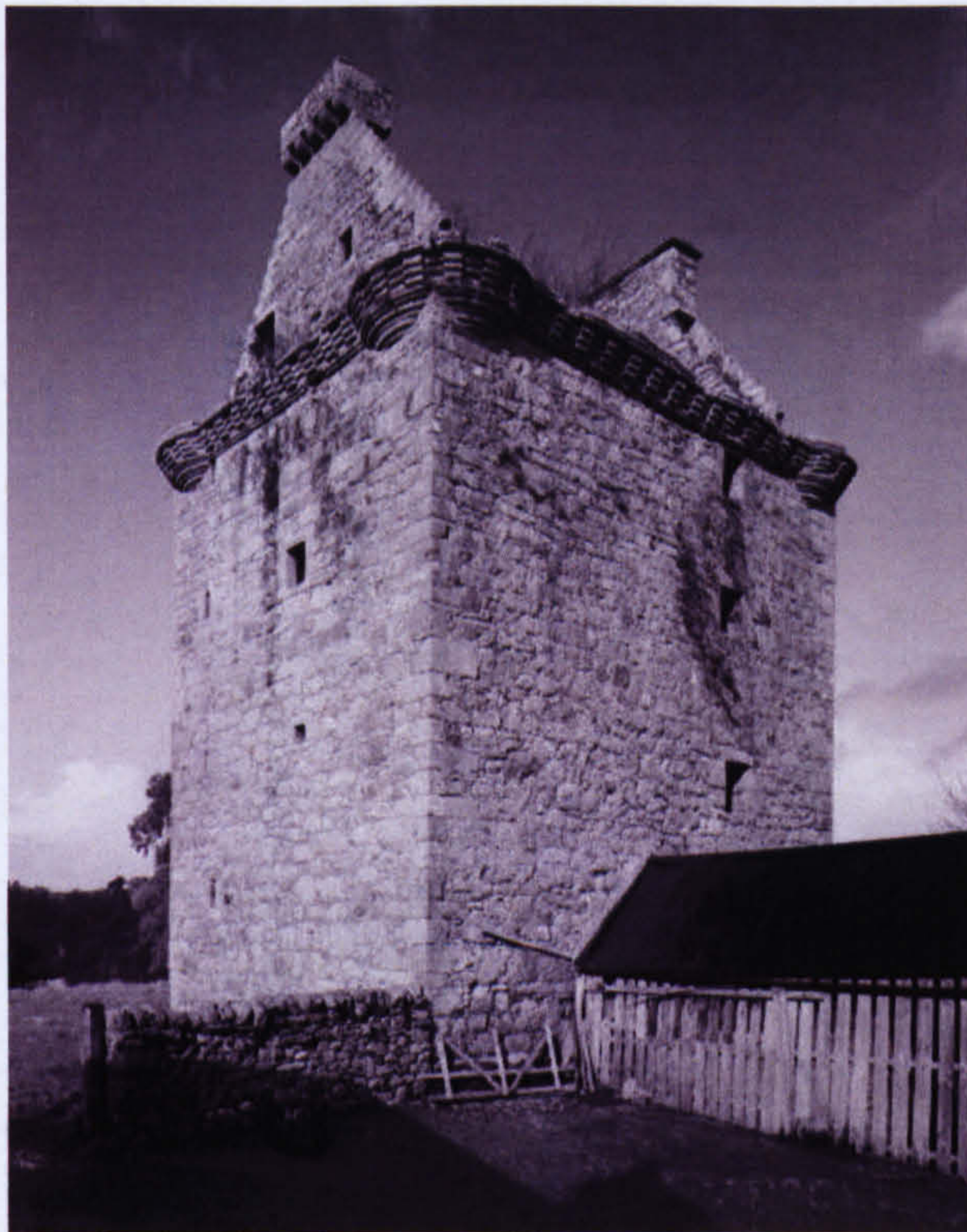
Fig. 2.2: Gilnockie Tower, Canonbie, Dumfriesshire.
