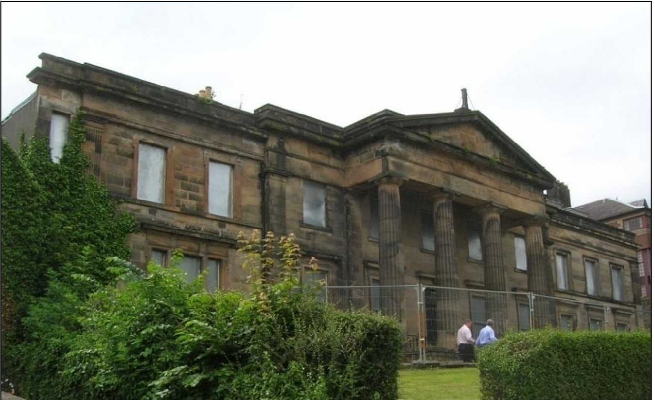
Figure 8: Commercial Bank, Spittal Street, Stirling. Built c.1827 by Alexander Bowie. Based on the valuation rolls of Scotland and the historical records contemporary with the construction of this building, A. Bowie was the operator of Thorneydyke Quarry. Bowie would probably have used the sandstone being extracted from his own quarry for the construction of this grand edifice.
