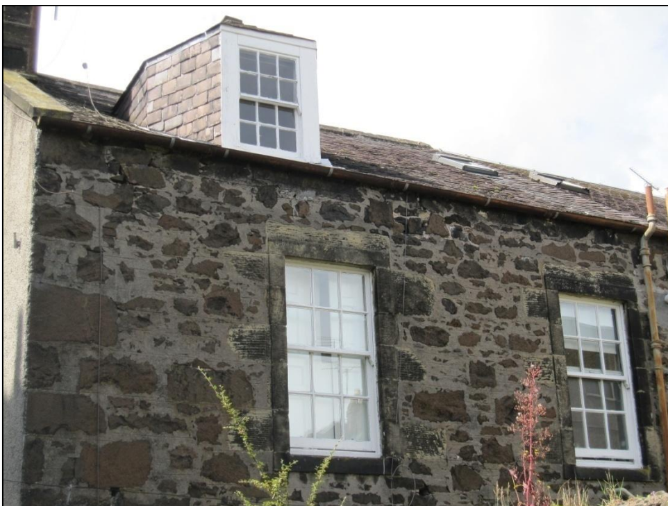
Figure 11: Rear rubble walling of building on Allan Park. Notice the different characteristics of the lesser quality local whinstone rubble walling, most likely extracted from the quarry across Dumbarton Road, versus the high quality ashlar and dressings used for the front facades of the Allan Park tenements (Figure 10).
