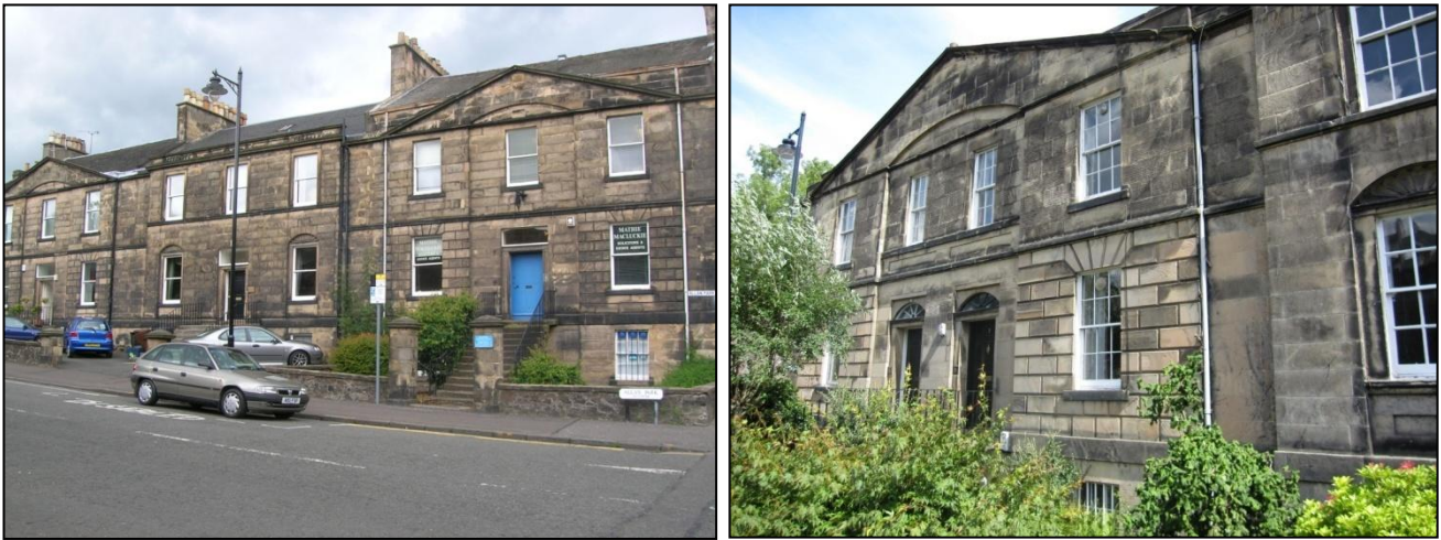
Figure 10: Allan Park, west (left) and east (right) side of road. Fourteen of the twenty-two houses on Allan Park were constructed by Bowie in the 1820s. It is highly likely that the tenements were constructed from Thorneydyke and Drumhead stone. Bowie's stone yard was located behind the west block of housing along Dumbarton Road. Stone from Thorneydyke Quarry (and possibly Drumhead Quarry) was stored and sold here.
