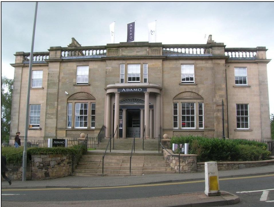
Figure 7: Front elevation of Craigs House, The Craigs, Stirling. Built c.1817 by Alexander Bowie, Stirling builder and operator of Thorneydyke Quarry. The sandstone may have been extracted from Thorneydyke Quarry, as Bowie was the builder and quarry operator. Further investigations would need to be undertaken to examine this possibility.
