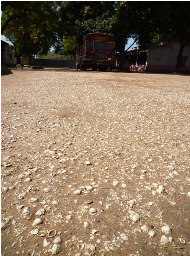
Figure 4. Cockle-shell road at the Gambian Technical Training Institute, The Gambia
