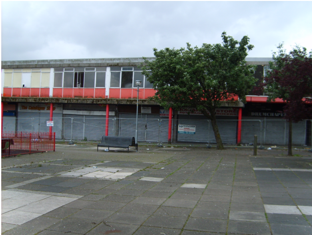
Figure 7.4 Interior of Drumchapel shopping centre
