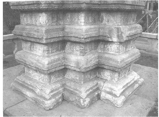
Fig. 30. Foundation of Wŏn'gak-sa pagoda.
