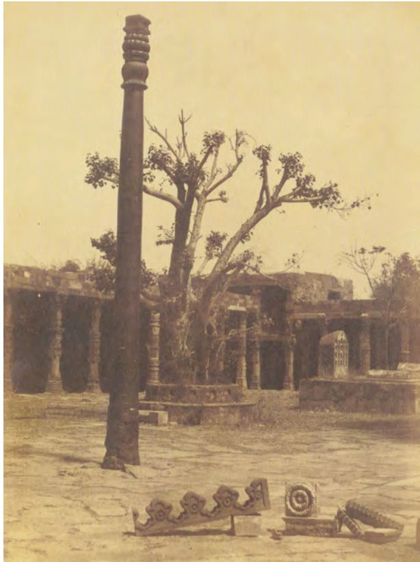
Fig. 1-18 Charles Moravia, Architectural fragments scattered around the Iron Pillar in the Qutb Minar Complex, Delhi , c.1858. As illustrated in Pelizzari 2003, p.38.
