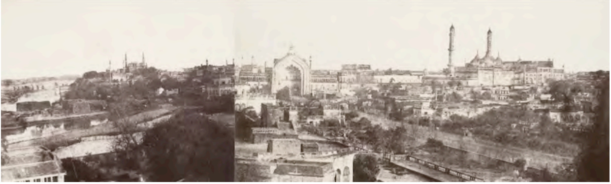
Fig. 2-2 Alexis de La Grange, Lucknow, The Rumi Darwaza, with the Asafi Imambara to the right and river Gomti to the left , 1849-51, two albumen prints. The Canadian Centre for Architecture, Montreal.
