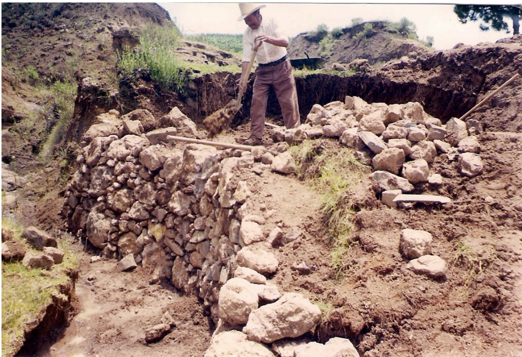
Infilling gullies and constructing stone wall
