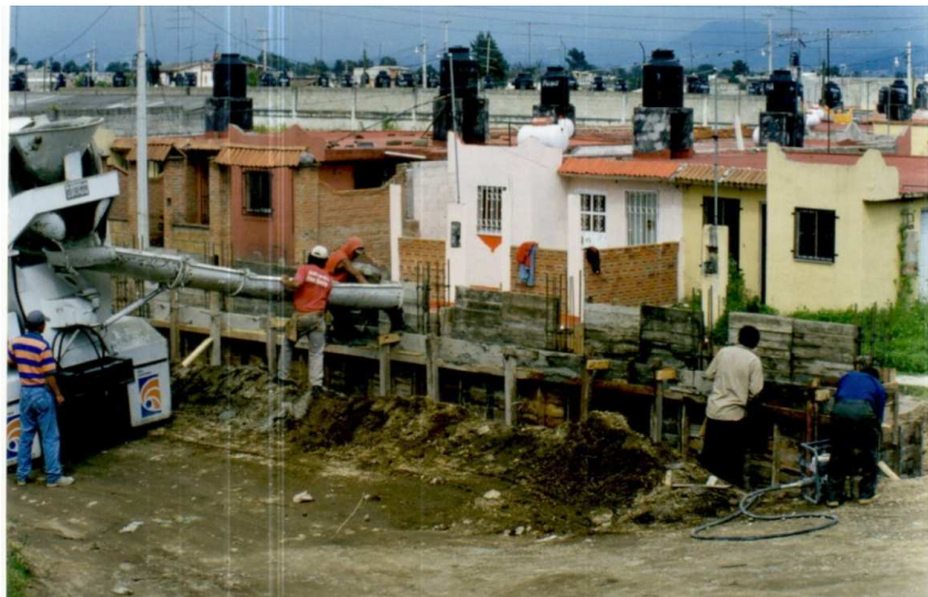
Figure 9 Locals at the EmC. Building the wall Source: EmC neighbour
