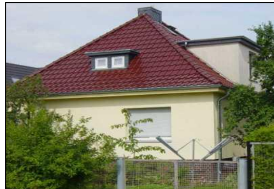
Picture 12: The same house after an illegal thermal renovation job, with 6 cm of roof insulation and 4cm of wall insulation.
