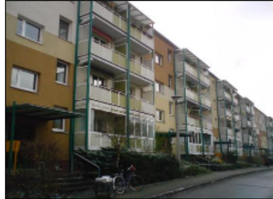
Picture 8: Decoupled balconies, added to a communist-era apartment block in Berlin. This method reduces heat loss.
