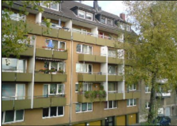
Picture 7: Apartment block with narrow balconies, which often become unusable when thick external wall insulation is applied.
