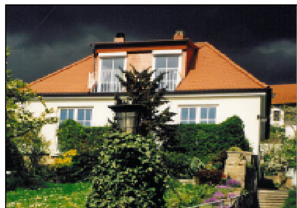
Picture 6: Würzburg house after thermal renovation.
