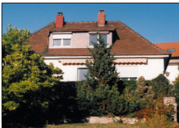
Picture 5: Würzburg house before thermal renovation. Note the large roof overhang.
