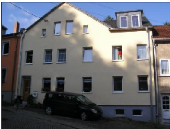
Picture 3: Illegally renovated house in Thüringen, below EnEV standards but far superior to most other houses in the street. 8cm of external wall insulation.
