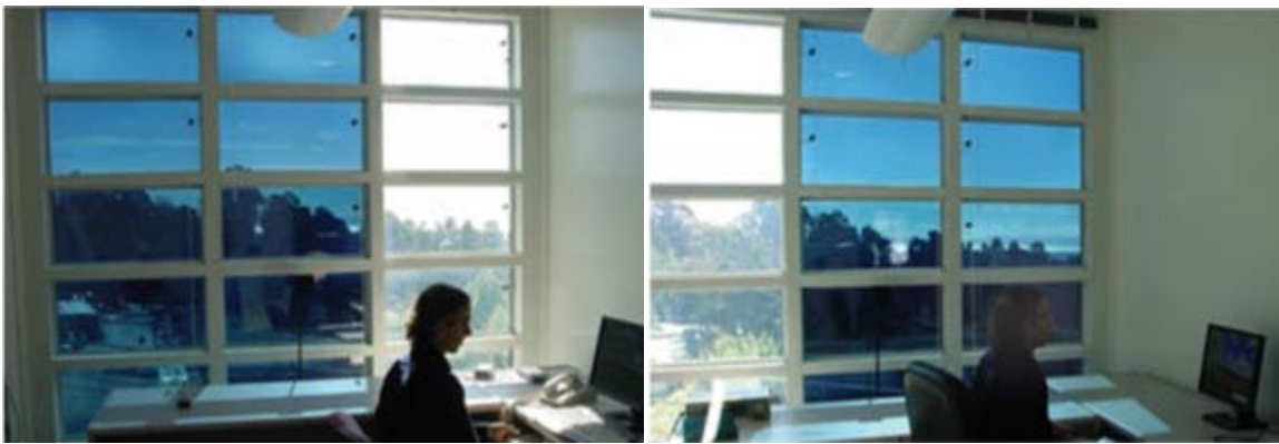
Figure B-4. Occupancy Comfort Study Allowing Users to Adjust Different Window Pane per User Comfort (Sage Electrochromic, 2006a).
