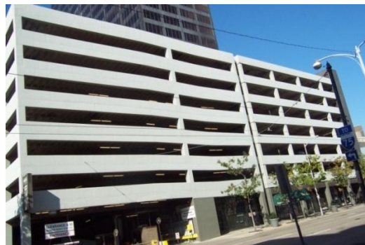
Figure 11. AMPCO Parking Garage, Dayton Ohio
