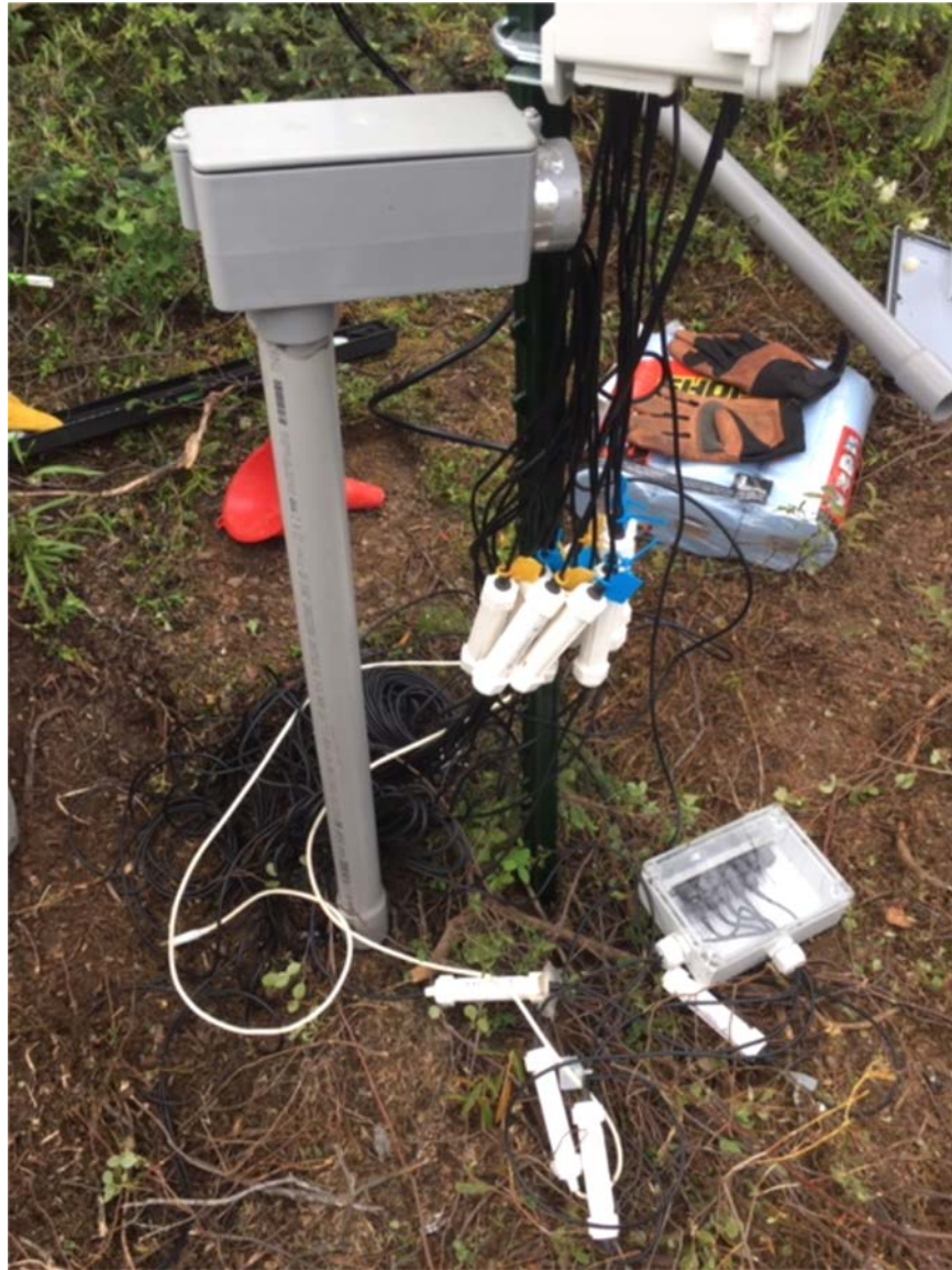
Figure 3.15: The Process of Upgrading Station Two
