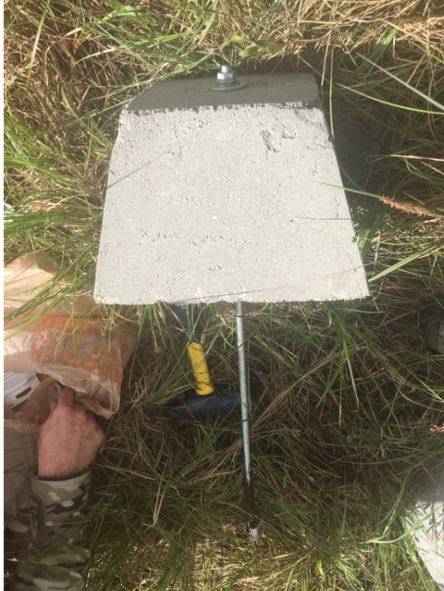
Figure 3.3: Completed Tripod Foundation
