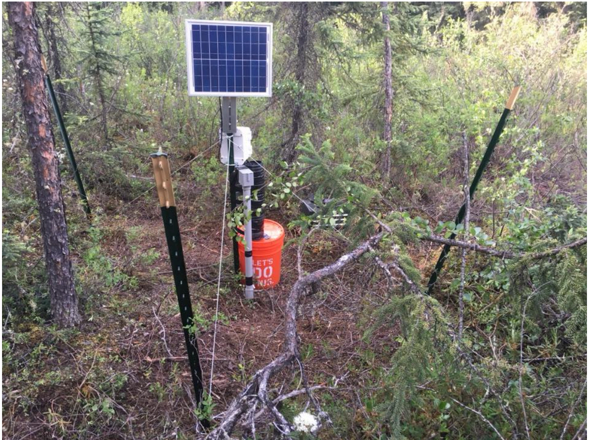
Figure 3.13: Station One Upgrades
