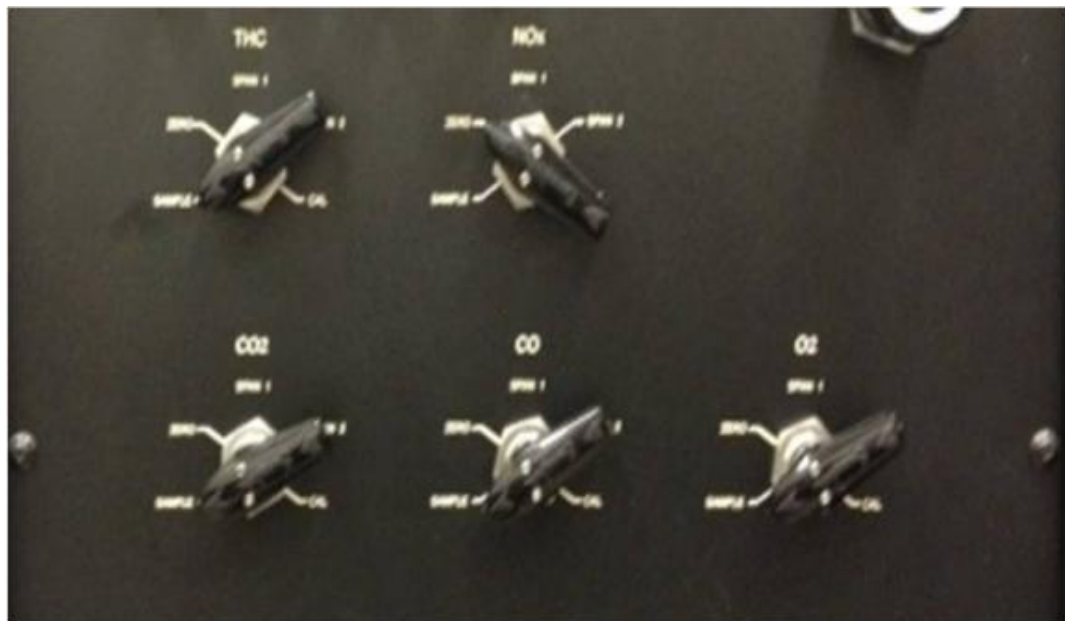
Figure A.5: CAI flow switch panel
