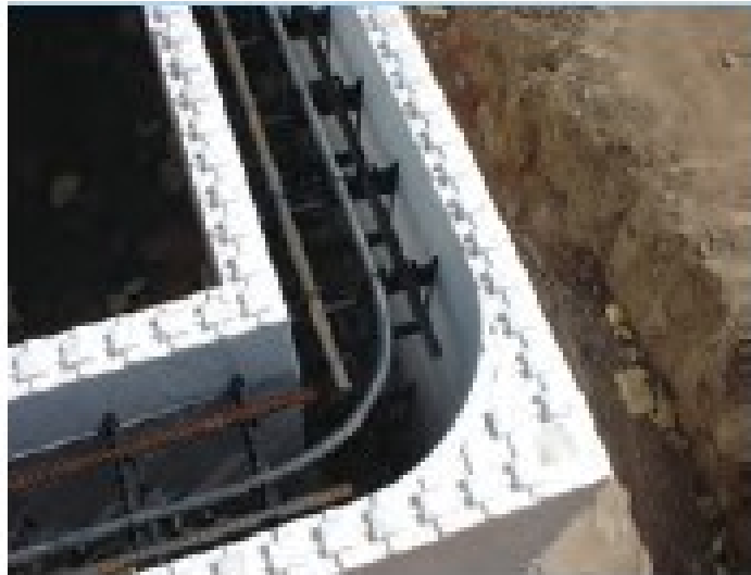
Figure 2. Insulated Concrete Forms with Rebar (ICF Photo Gallery, 2013)
