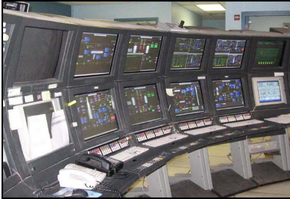
Figure I-1 BP Texas City Control Room Layout Representative of a typical centralized process control room layout consisting of multiple displays to monitor remote processes. (U.S. Chemical Safety and Hazard Investigation Board, 2007)
