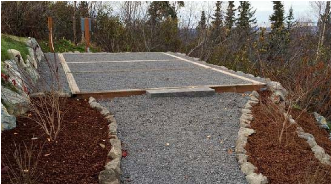
Figure 7. Gravel Pad Foundation (Cedar Built, 2015)
