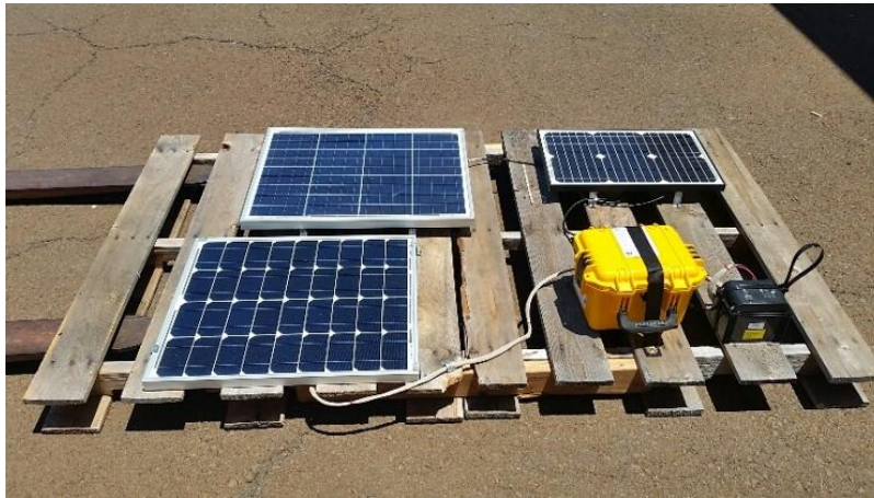
Figure 22. Complete test system with battery and charging panel
