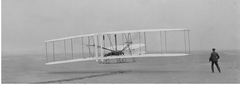
Figure 7. Orville Wright at the Controls as Wilbur Runs Alongside [16]
