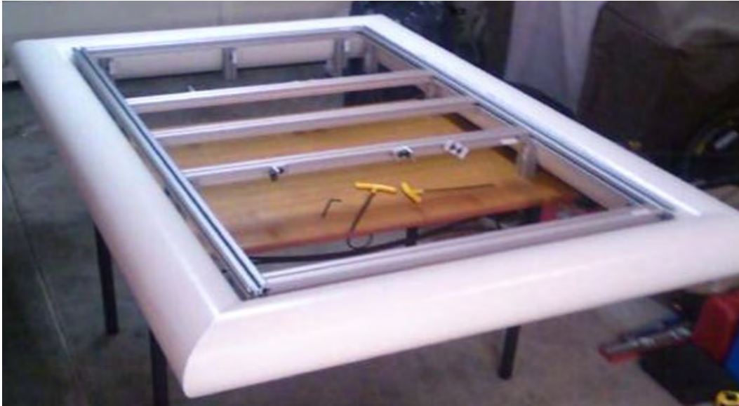
Figure 41: Bottom Plate Frame with PVC Pipes Installed
