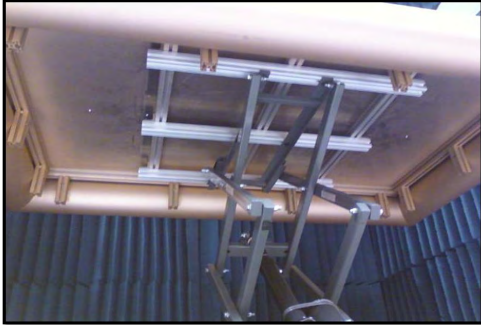
Figure 56: Bottom Plate Installed on Scissor Lift
