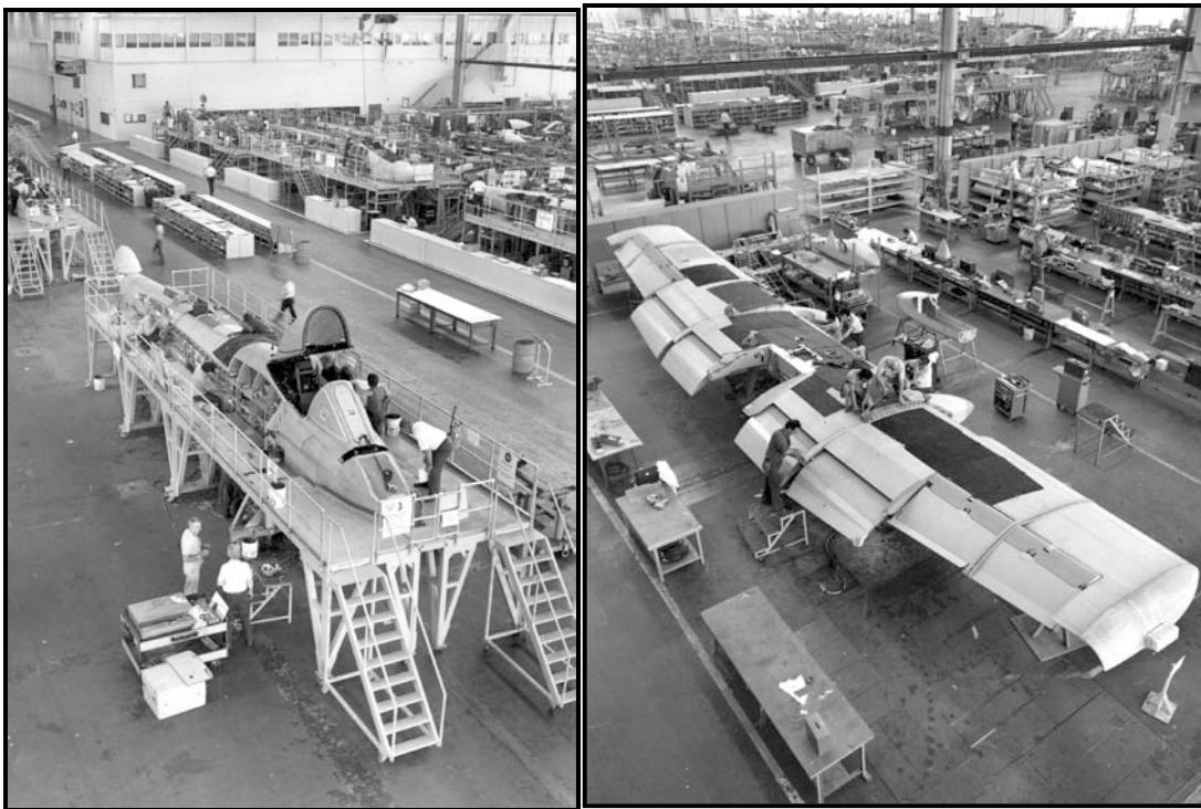
Figure 19. A-10 Fuselage and Wing Production
