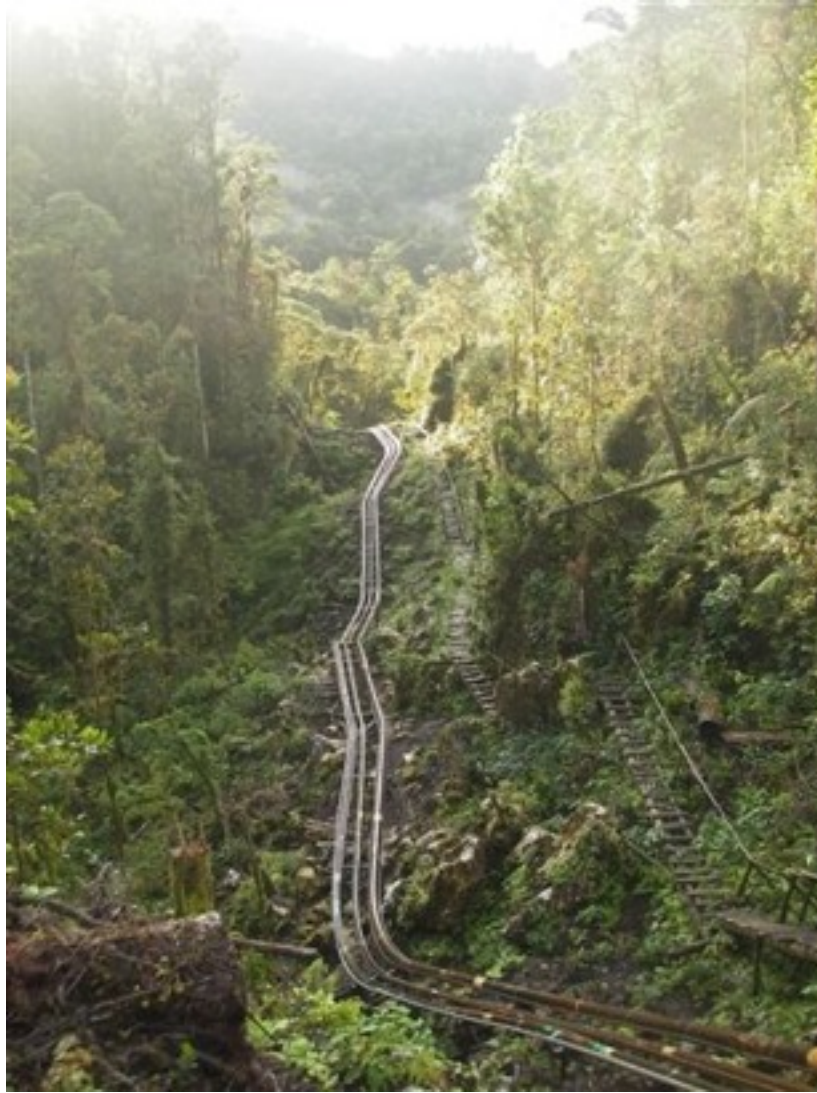
Fig. 5 Oil Pipeline through the Rain Forest (Courtesy of OSL)
