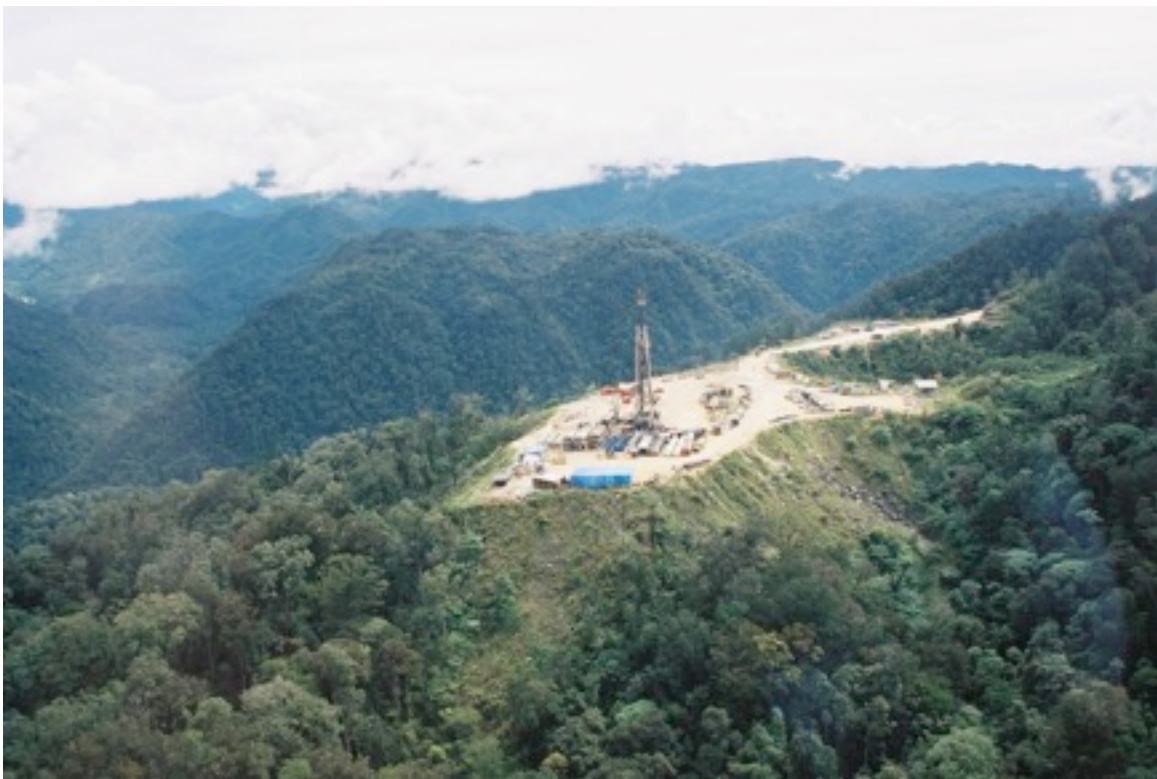
Fig. 9 Well-Head at Moran (Courtesy of OSL)
