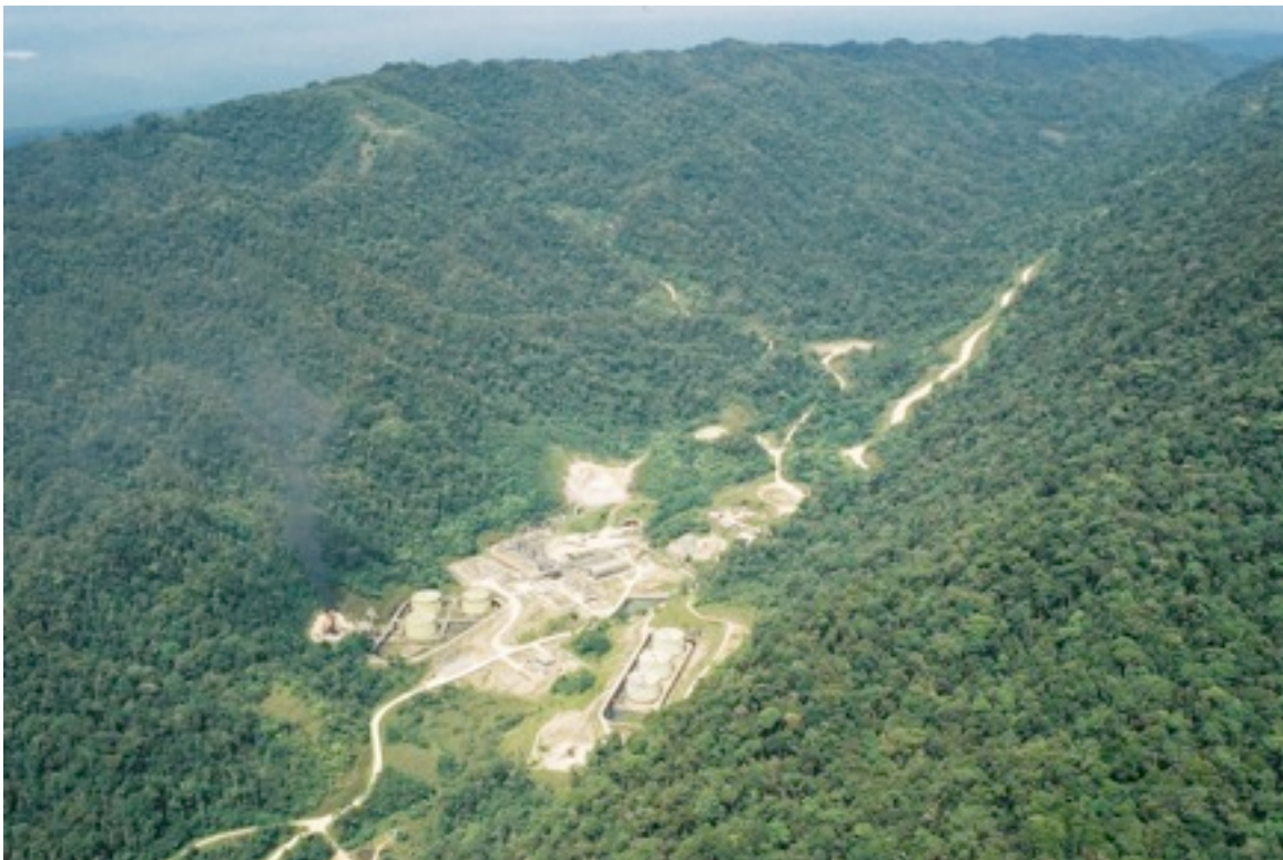
Fig. 7 Central Production Facility from the Air (courtesy of OSL)
