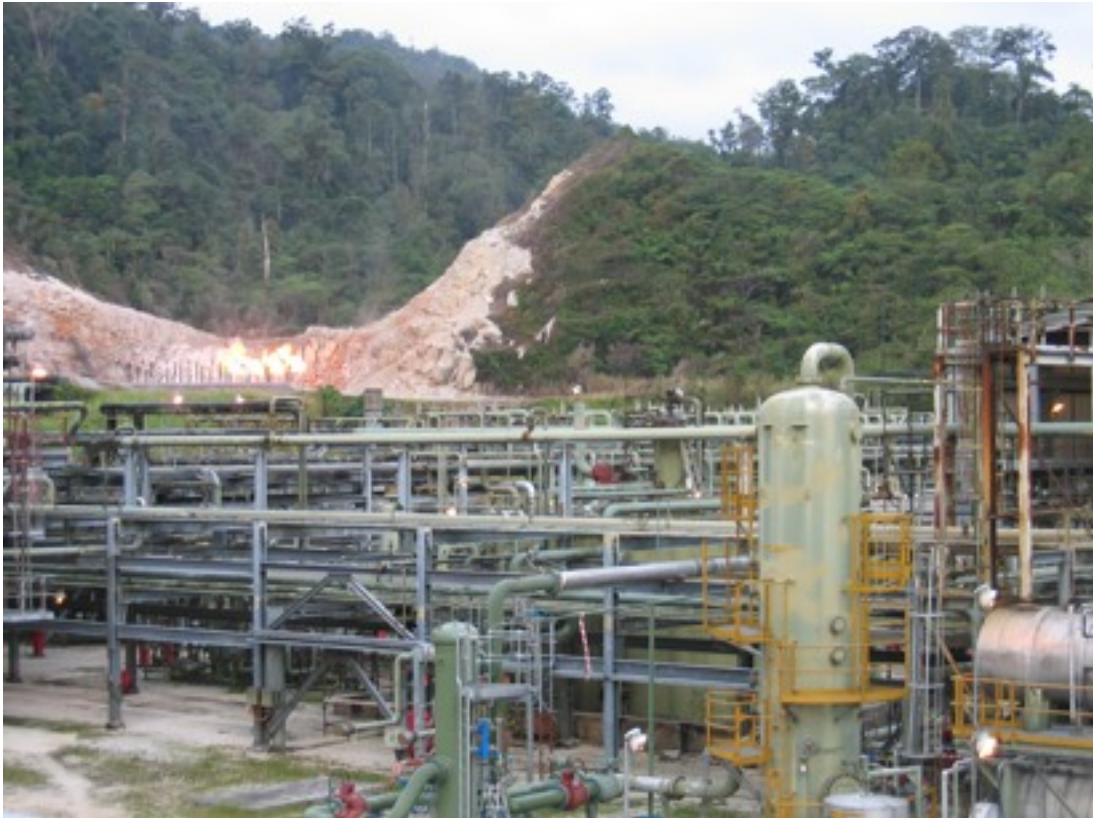
Fig. 8 Central Production Facility from Ground (courtesy of OSL)
