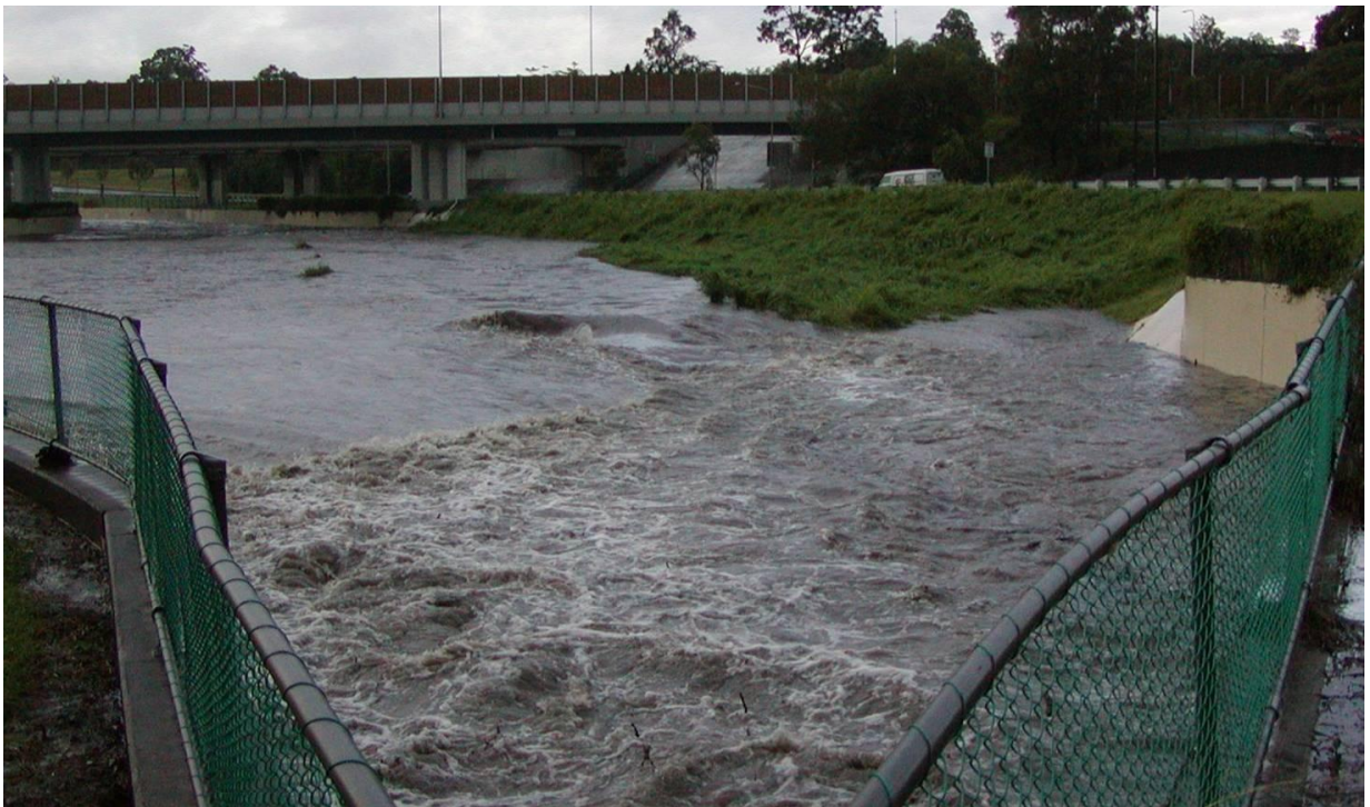
Figure 1.16 Sediment laden flow passing through a hydraulic jump. Flow through culvert MEL-C-3 of Norman Creek underneath Ridge Street, Brisbane, Australia in flood on 31 December 2001 around 6:10 am at the end of a rainstorm. Photograph courtesy of Hubert Chanson.
