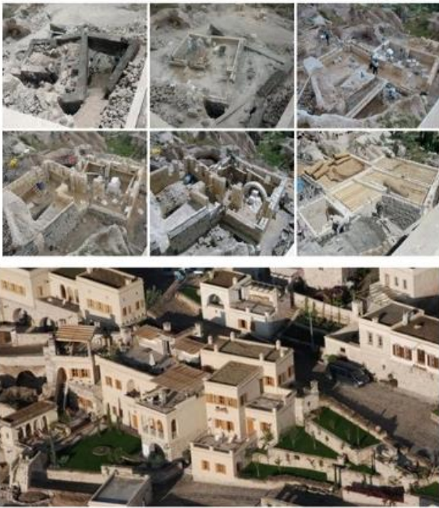
Figure 5. Restoration of Vernacular Housing Consulted by Cansever for Argos (URL 8).
