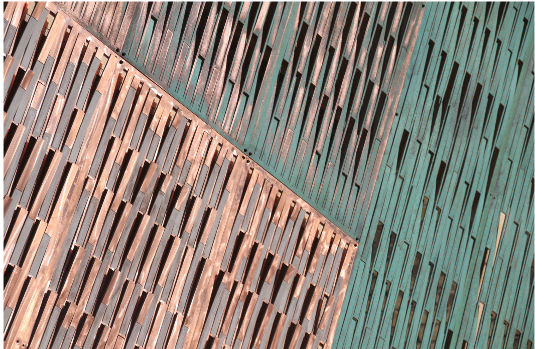
FIG. 3 Sense Envelope III. Copper and polypropylene are forming a thermally active composite. Design/fabrication by Isak Worre Foged and Anke Pasold. Photograph by: Isak Worre Foged.
