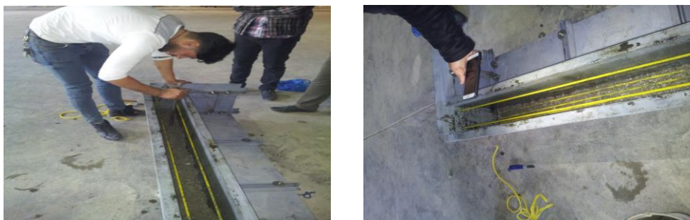
Plate 1. Steel mold used and concrete casting process
