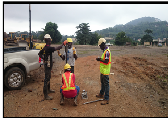
Figure 3. Dynamic Cone Penetration Tests at the Project Site. Source: Authors, 2015
