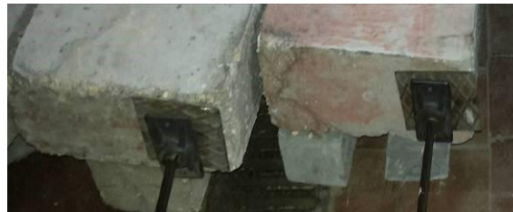
Figure 5. Anchorage zone of the tested prestressed concrete beam
