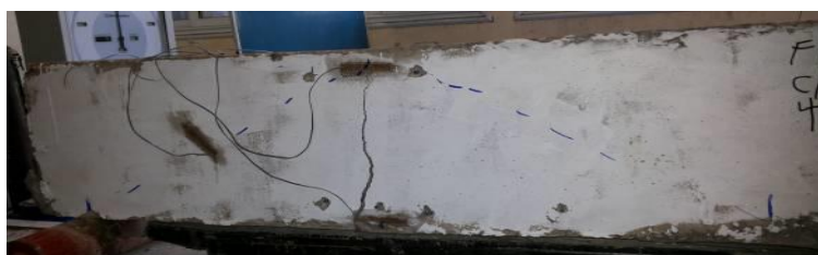
Figure 18. Crack Pattern and Mode of Failure of the fully prestressed beam with CNT under Elevated temperature (FP –CNT-400)
