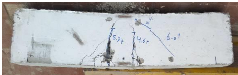
Figure 12. Crack pattern and mode of failure of a non-prestressed beam with CNT (RC- CNT)
