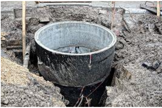
Figure 1. Cylindrical concrete well environment
