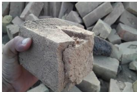
Figure 2. Defective brick sample
