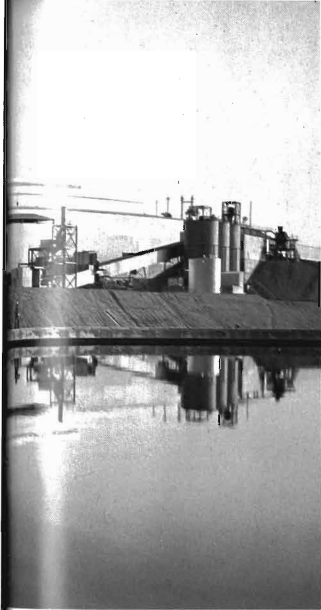
One of four 325-ft thickeners reflects the Phelps Dodge Tyrone concentrator building in its settling pool. Photograph by Ray Manley.
