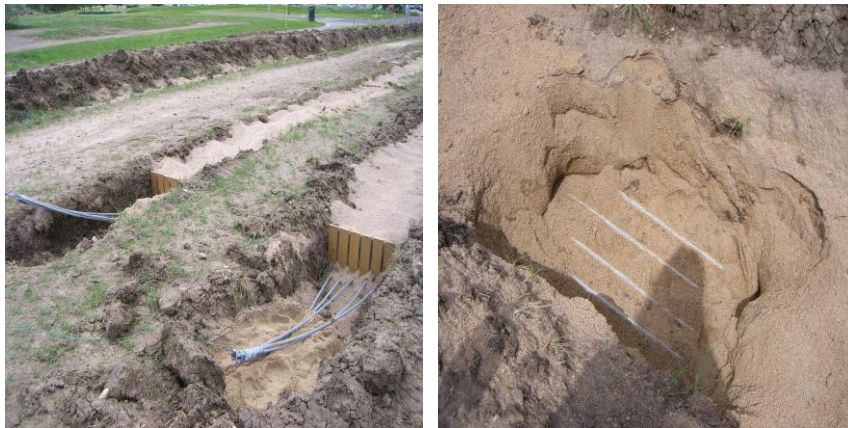
Fig. 11. (Left picture) Ends of two anchors extending from trenches 1 (left) and 2 (right), 7' apart. This shows the plywood spacers used to hold the strands approximately 4" apart in the trenches, as shown in the right photo. © 2009 IEEE. Reprinted, with permission, from 39.
