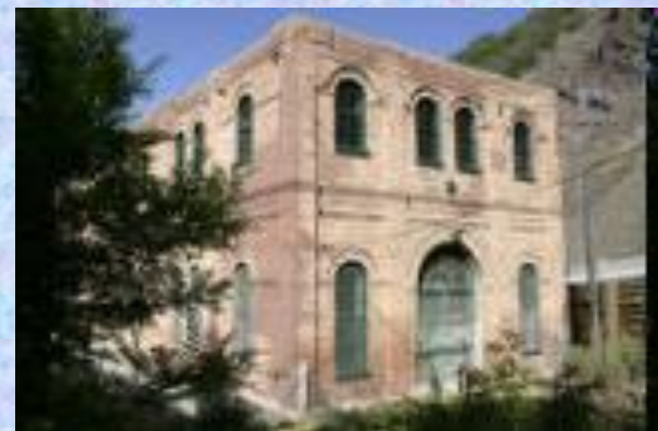
[1895 Stairs Hydroelectric Power Station]
