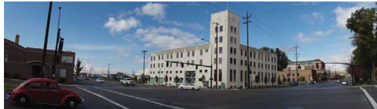
400 S and 400 W. Site is on left, Big D building on the right.
