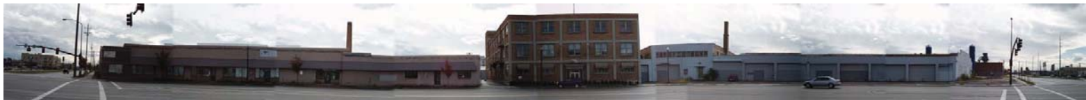
North elevation of the existing block.
