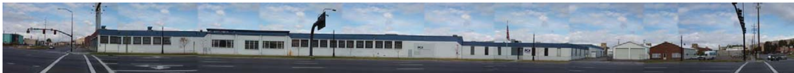
South elevation of the existing block.
