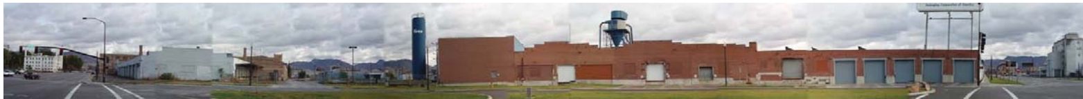
West elevation of the existing block.
