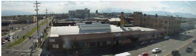
NE corner of site from above.
