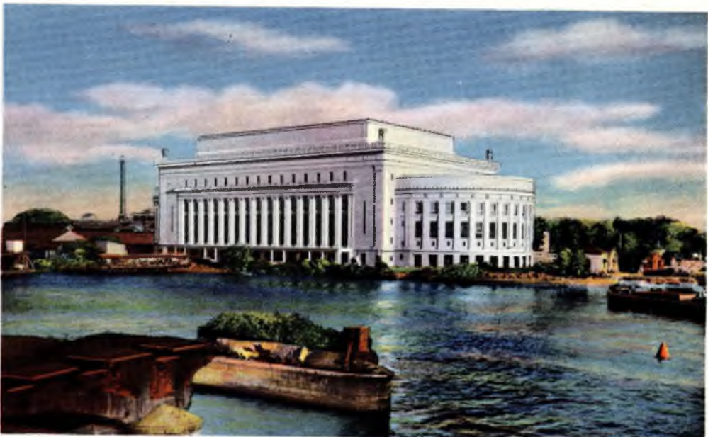
MANILA'S NEW POST OFFICE FROM PASIG RIVER
