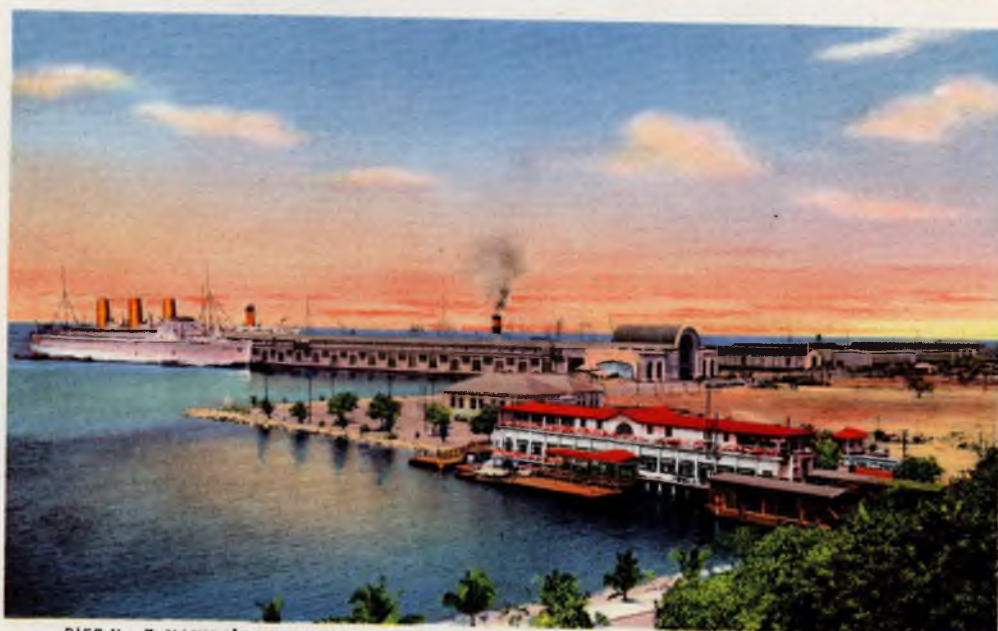
PIER No. 7, MANILA'S NEW PIER
