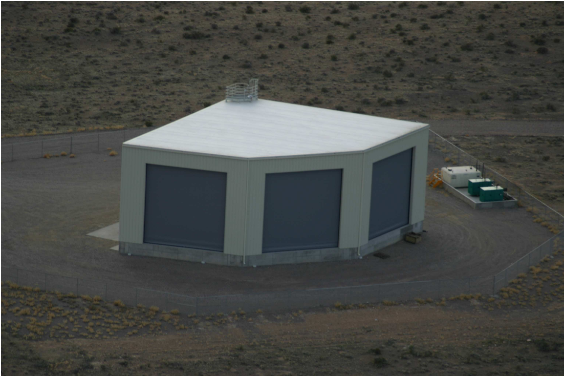
Figure 3.7: Aerial photograph of the Long Ridge telescope building.
