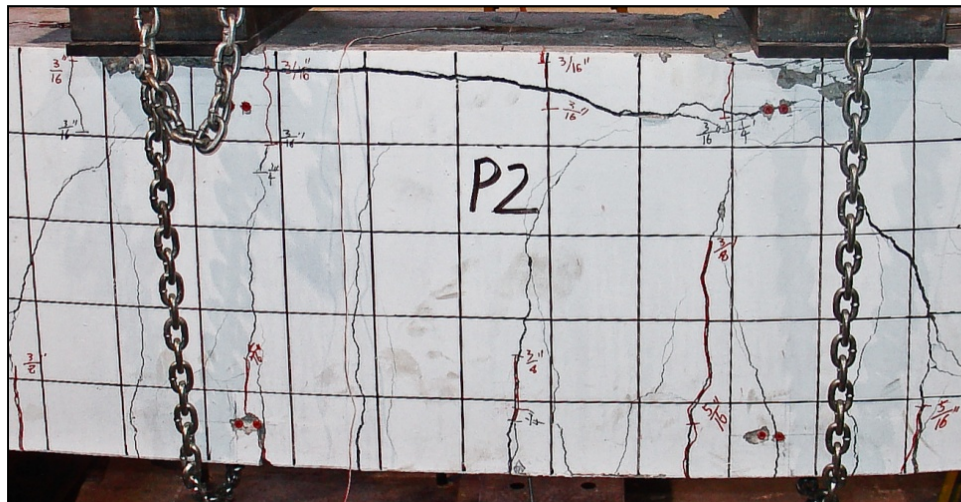
Fig. 5.6 – Failed specimen P2 (control), Grid = 4" (100 mm)
