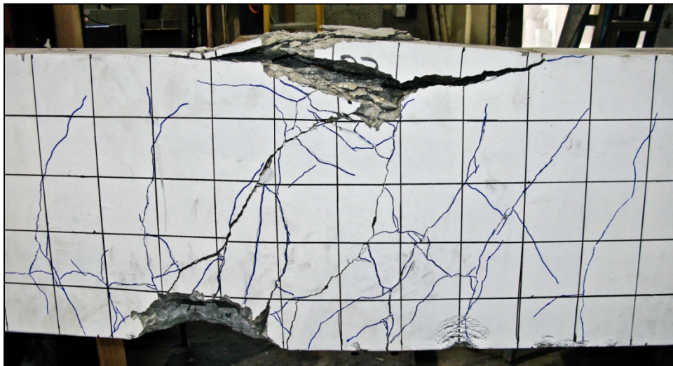
Fig. 5.8 – Failed specimen RP3 (repaired), Grid = 4" (100 mm)
