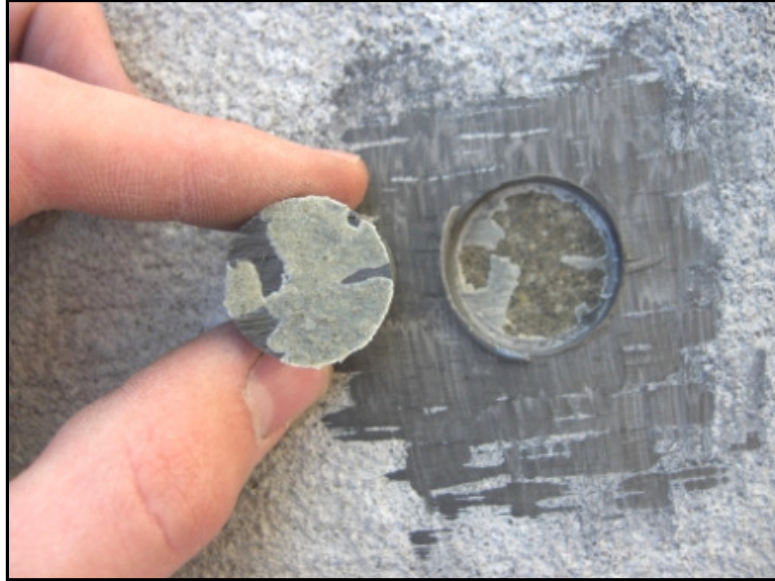
Figure 4.22: Original concrete region bond test
