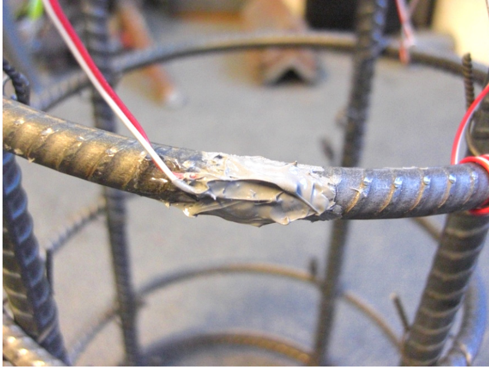
Figure 2.13: Internal strain gauge protective coating
