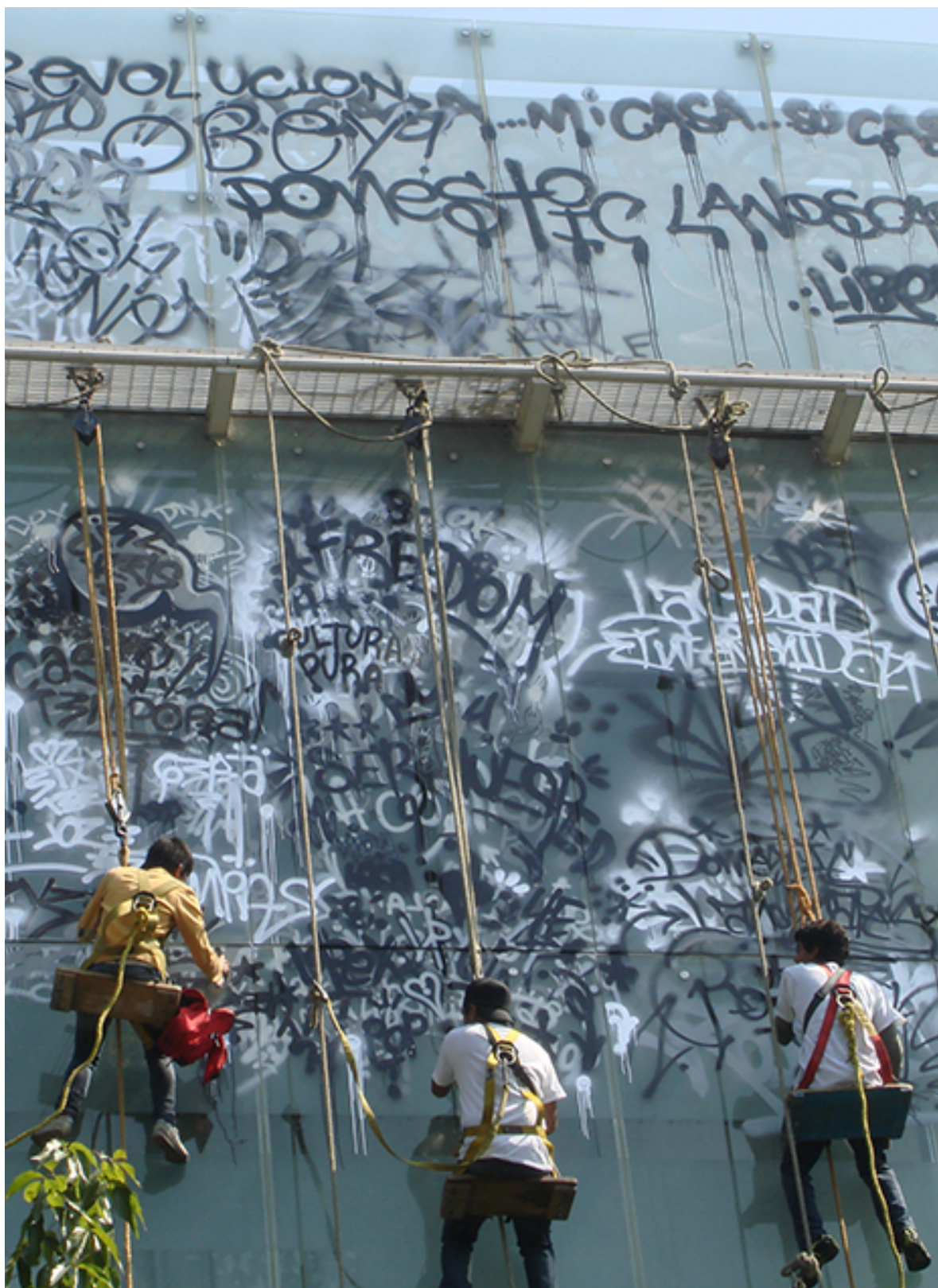
Figure 14. Installation of Habita intervenido
