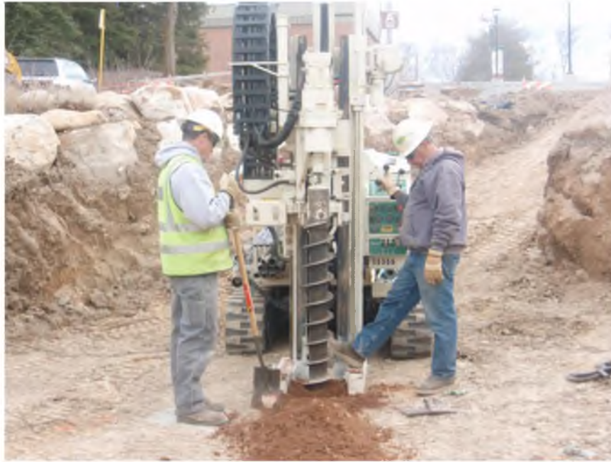
Figure 53. Photo of Well Drilling
