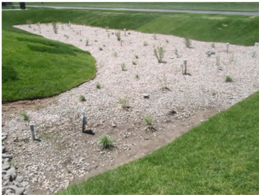
Figure 56. Photo of Completed Mountview Park Bioretention Cell
