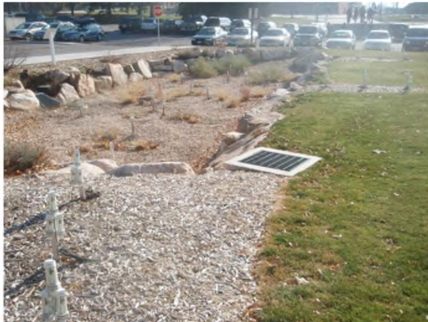
Figure 54. Photo of Completed SCIF 4 Bioretention Cell
