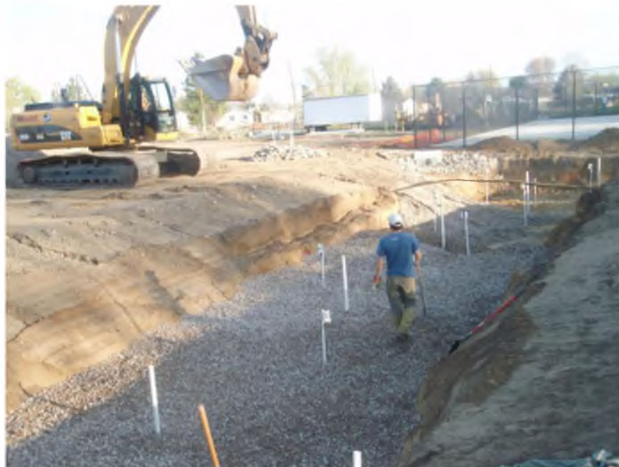
Figure 55. Photo of Construction at Mountview Park
