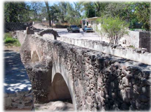
Figure 5. Aqueducts, Tecozautla, Hidalgo, 2006.
