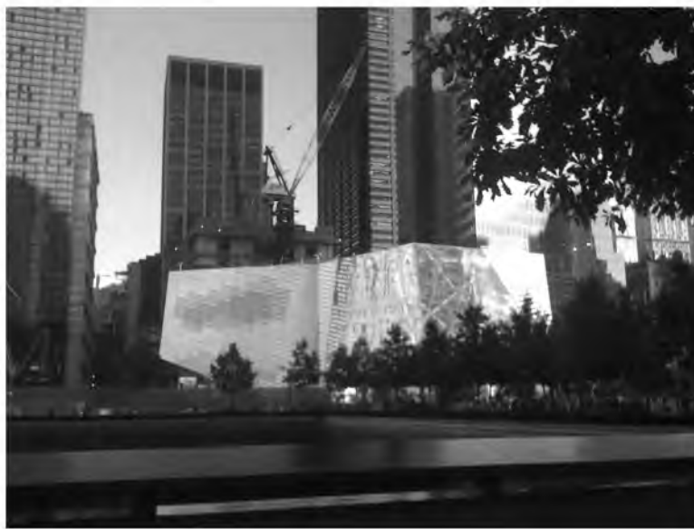
Figure 13: Museum Building at the 9/11 Memorial
