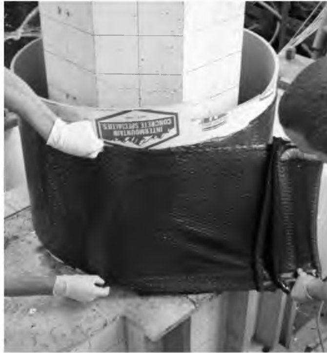
Figure 89. Applying Additional Layers to CFRP Shell
