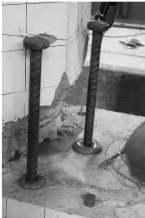
Figure 87. Epoxying of Headed Bars
