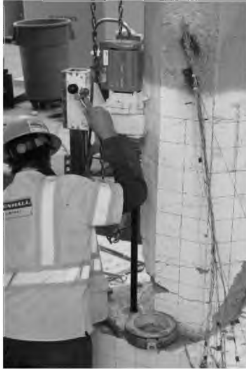
Figure 86. Drilling of Postinstalled Head Bar Holes
