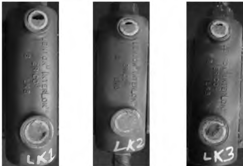
Figure 19. Void at Top of Splice Sleeve
