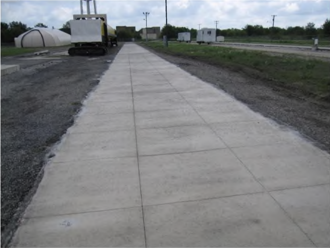
Figure 4.1. Constructed full-scale thin FRC overlay, view of section 1.
